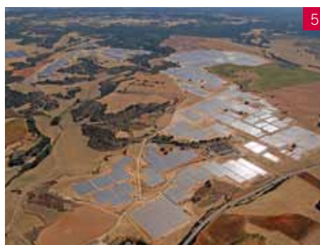
5. NOBESOL PV array at Olmedilla de Alarcón (Spain) 60 MWp (452 INGECON® SUN Power)
