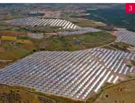
FRV 2. Royalla Solar Farm (Australia) 20 MW (10 INGECON® SUN PowerStation)
